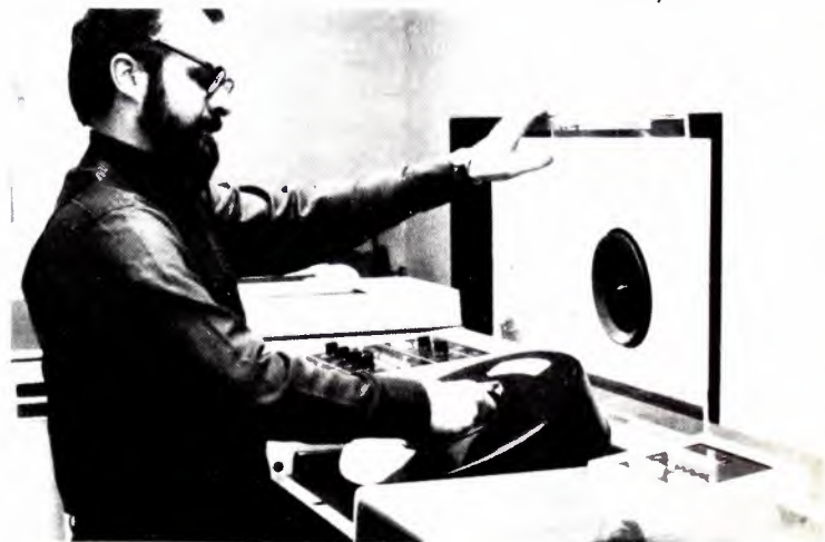
The magnetic disc files of the NCR Century 100 computer, which hold 8.4 million characters of data, provide a random-access store of information from which Star Stations produces logs, availability listings, and affidavits, and from which they are able to do bookkeeping and billing and a number of timely management reports.
